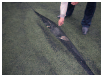
A pitch with open seams is not safe to play on and can cause injuries
